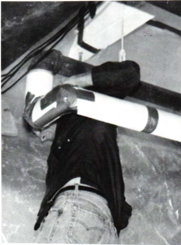
Tom Botts, a worker for Crossland Construction, checks the wiring of a hall light in Dyer.
