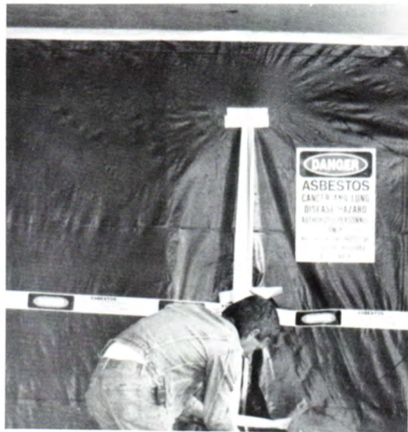
Danny Frost, of Crossland Construction, finishes taping up plastic before completing asbestos removal.
