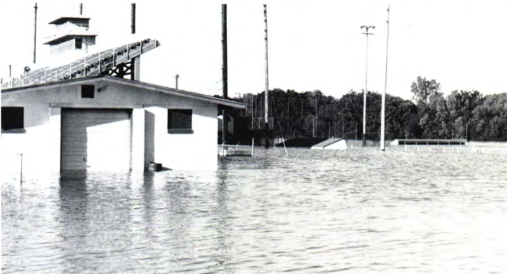
Flood water engulf the maintenance department during the September high water.
