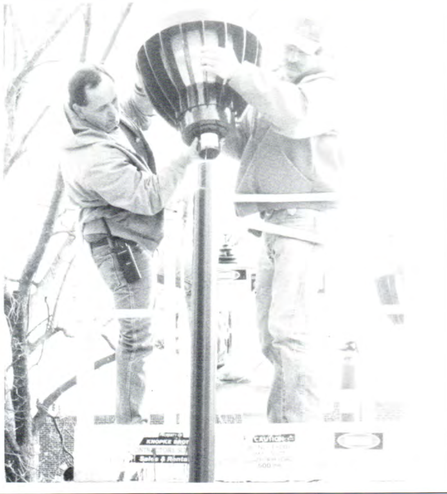
Electricians Toby Woodworth (left) and Don Fields install the heads on lamps that extend from Shipley Hall to I Street.
