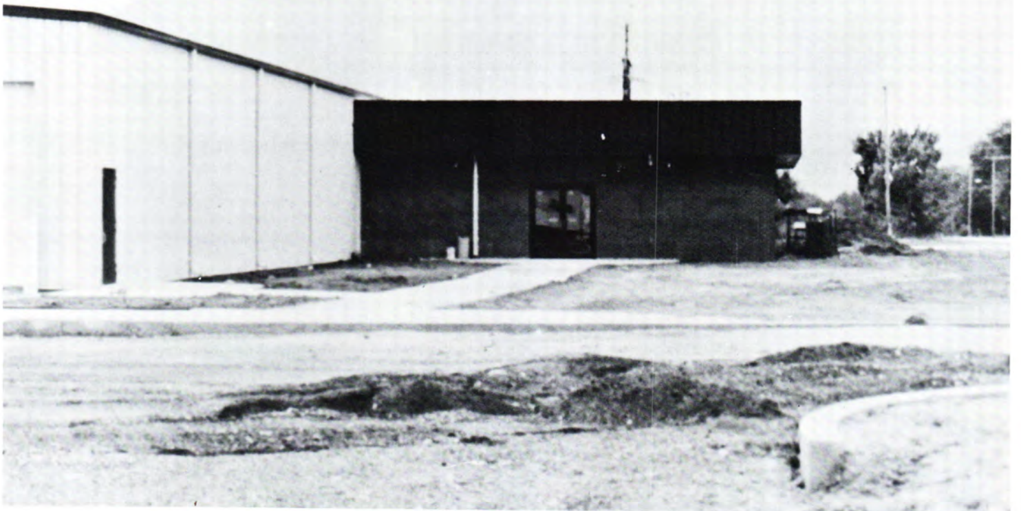
The new multi-purpose Equine Center area was near completion during the grand opening in December. The Equine Center will be utilized by both the college and various community groups.
