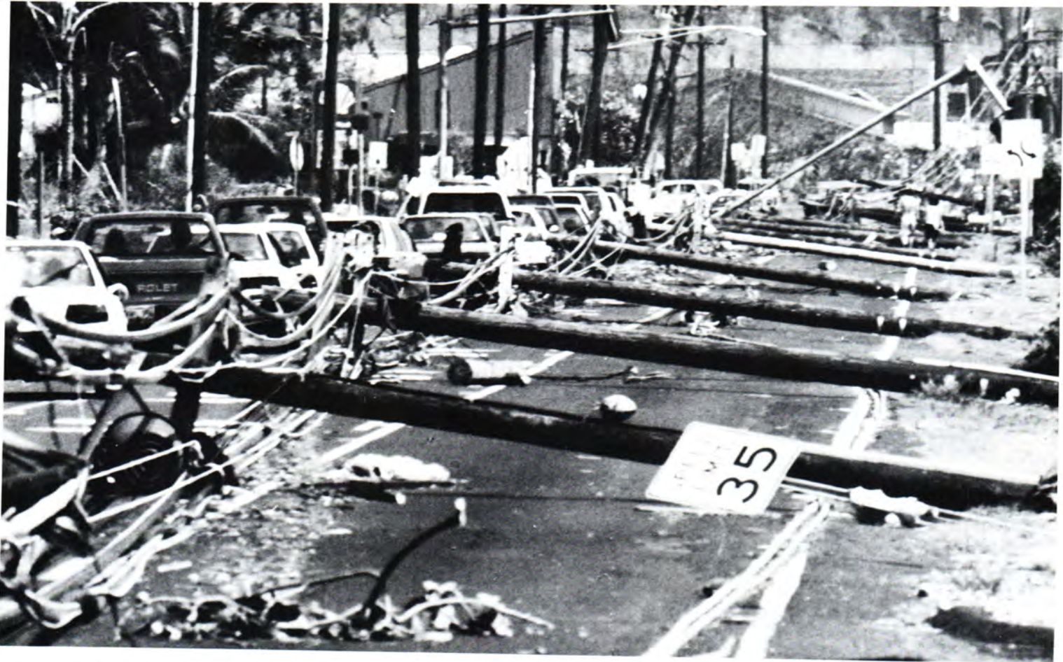
Telephones poles lined the streets after Hurricane Andrew slammed into the coast of southern Florida on Aug. 24, 1992 with winds gusting at more than 164 miles per hour.
