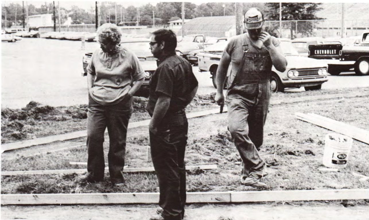
Maxine Edwards views sidewalk construction near the childcare center.
