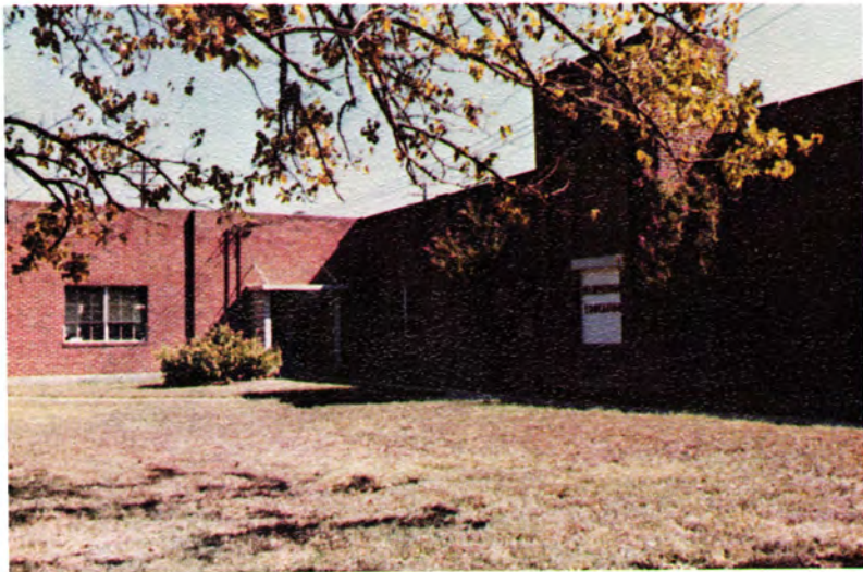
Ables Hall houses drafting and design, woodworking, automotive technology, general physical science, machine tooling, air conditioning, welding, electronics, and nursing.
