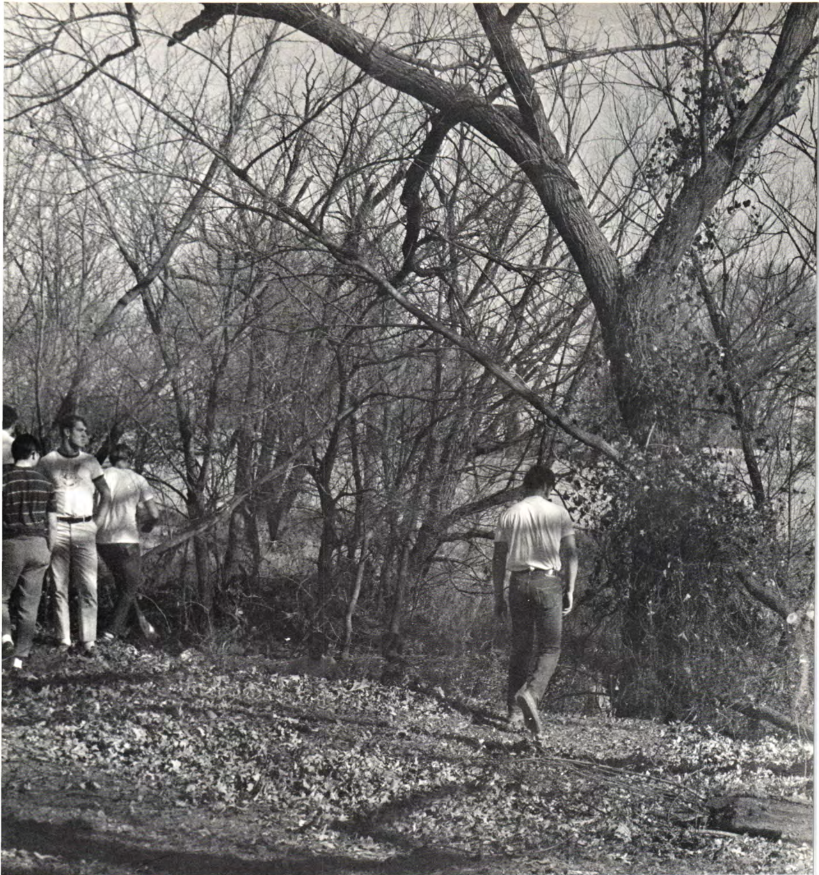
Student—faculty labor combined to fulfill the idea created by the Inter-Dorm Council to provide a recreational area east of the main campus near Tar Creek.
