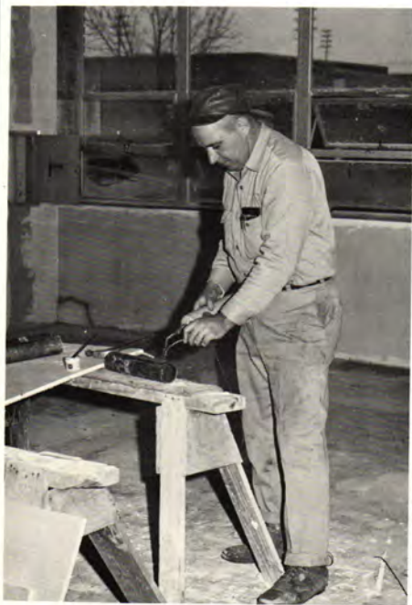
Renovation of Shipley Hall was inclusive of all facilities.
