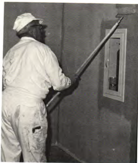
Final touches are being made in the renovation of Shipley Hall.
