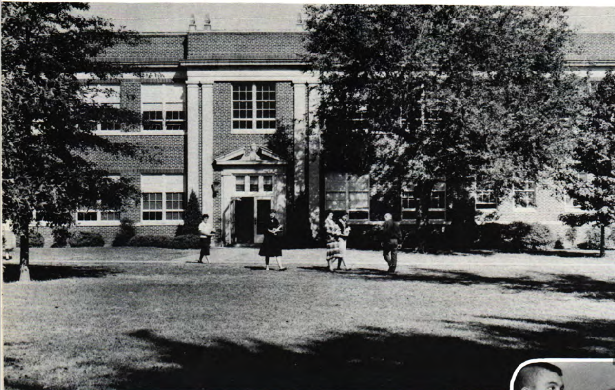
The Life Science building houses the Agriculture, Science, ROTC, and Electronics departments. The two story building is located on the north end of the campus. Below a Northeastern A&M student works on a chemistry project during an afternoon lab.
